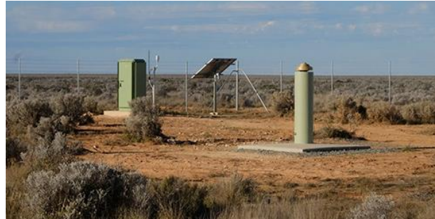
An Australian GNSS monitoring station
